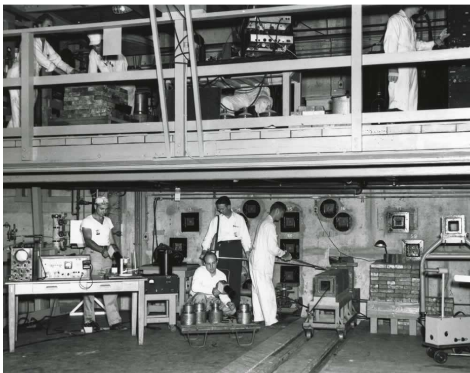
The side of the Graphite Reactor where the isotopes were inserted and removed to produce radionuclides for nuclear medicine and other research purposes
